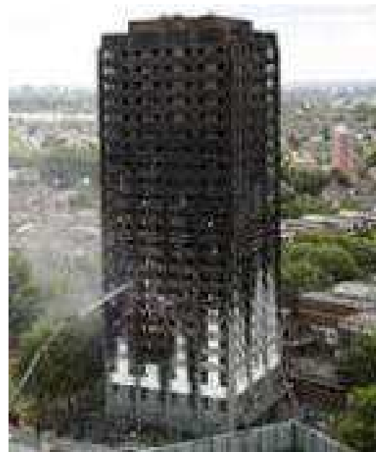
Grenfell Tower, UK (lipanj, 2017)
